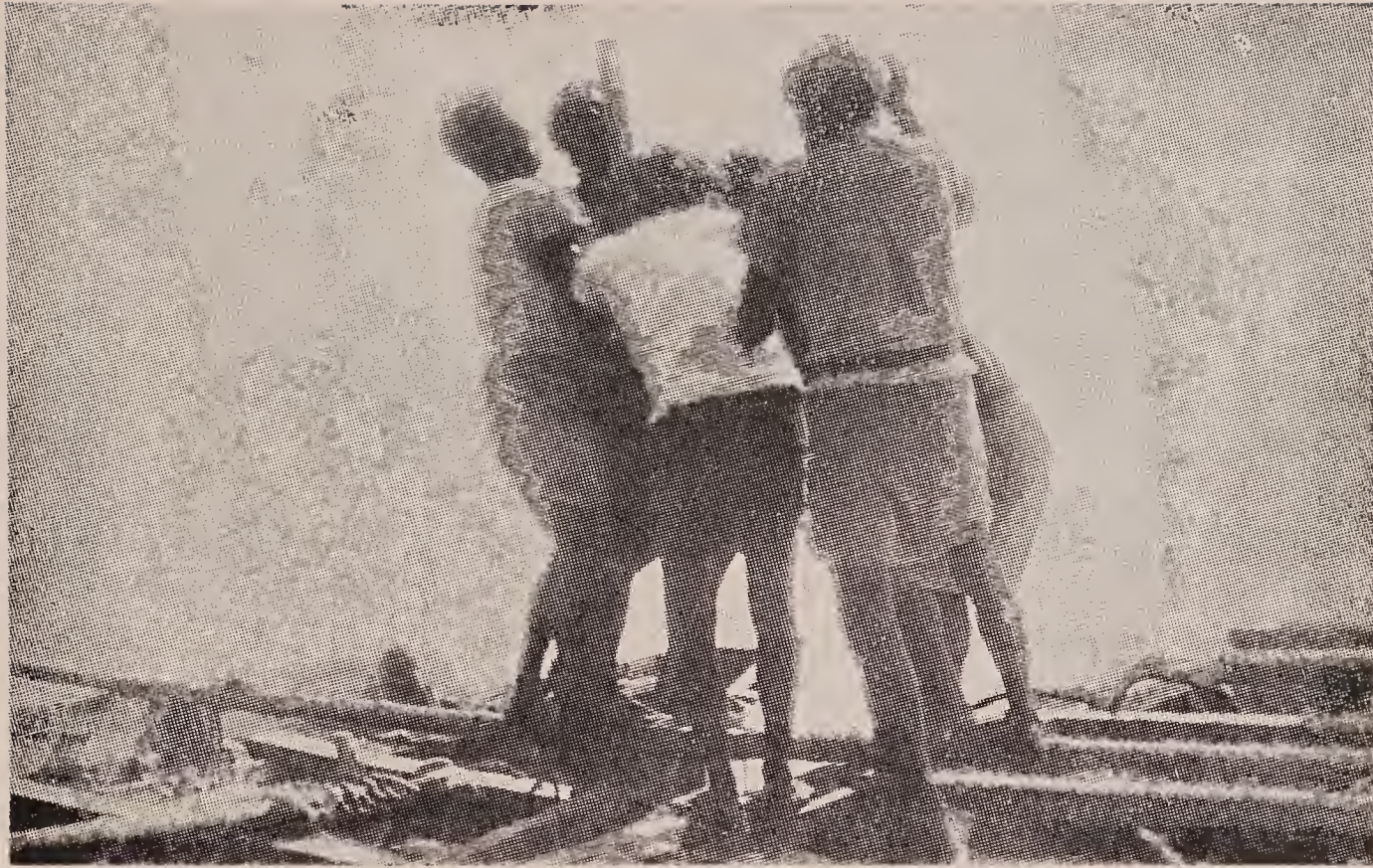
Planting of wooden posts to set the net
